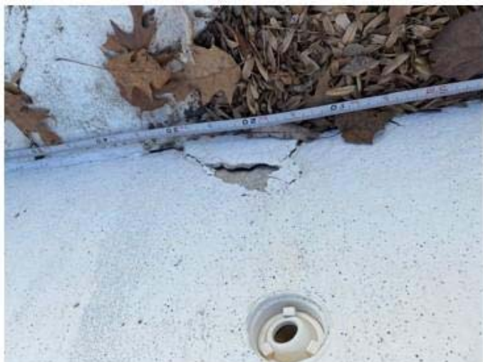
F. Special Construction - LLWP Pool Basin
